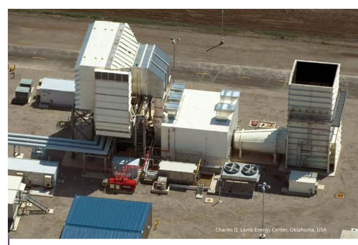
SGT6-2000E Heavy-duty gas turbine Power generation: 119 MW
