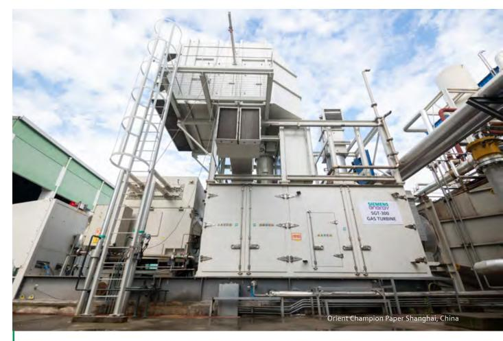
SGT-300 Industrial gas turbine Power generation: 7.9 MW(e) Mechanical drive: 8.4 – 9.1 MW The **SGT-100** industrial gas turbine is a proven unit for all electrical power generation and mechanical drive applications. The compact arrangement, on-site or off-site maintainability, and inherent reliability makes it an ideal gas turbine for the demanding **oil and gas industry**.
