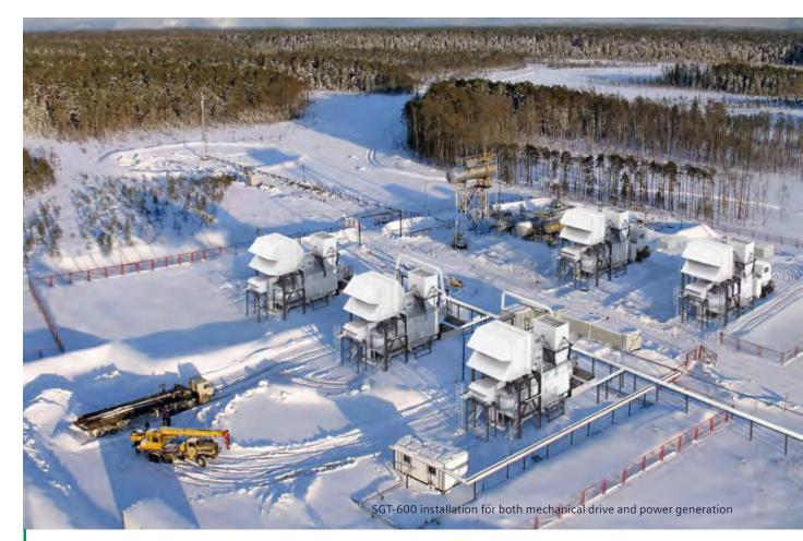
SGT-600 Industrial gas turbine Power generation: 24.5 MW(e) Mechanical drive: 25.2 MW The **SGT-400** is a twin-shaft gas turbine available in different configurations and power ratings to support power generation and mechanical drive applications from 10 - 15 MW. The twin-shaft arrangement allows for commonality of parts in mixed-duty installations.
