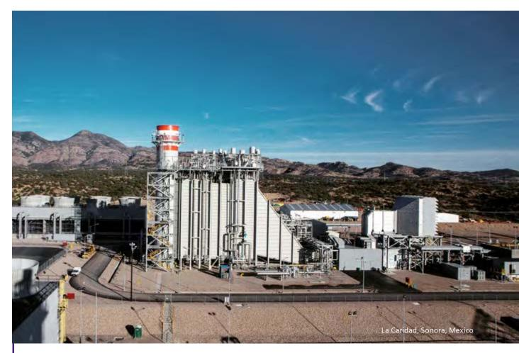
SGT6-5000F Heavy-duty gas turbine Power output: 260 MW
