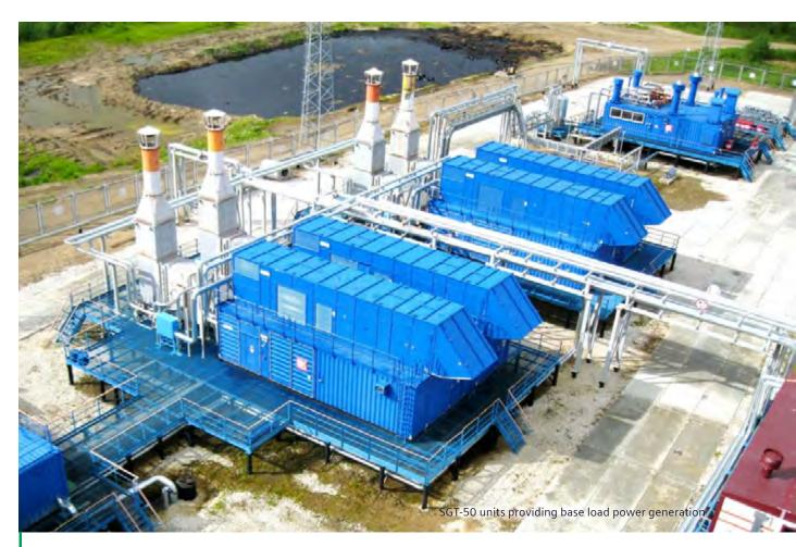
SGT-50 Industrial gas turbine Power generation: 2 MW(e)
