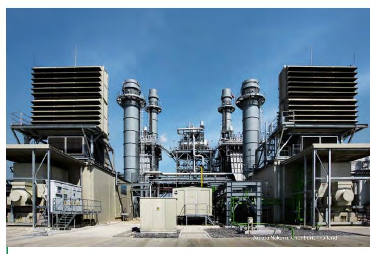
SGT-800 Industrial gas turbine Power generation: 45.3 – 62.5 MW(e)
