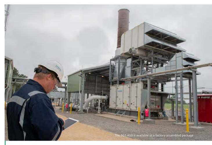
SGT-400 Industrial gas turbine Power generation: 10.5 – 14.3 MW(e) Mechanical drive: 10.9 – 14.9 MW The **SGT-300** industrial gas turbine has a rugged industrial design that enables **high efficiency**, **reliability**, and **excellent emissions performance** in a broad spectrum of applications for both power generation and mechanical drive.
